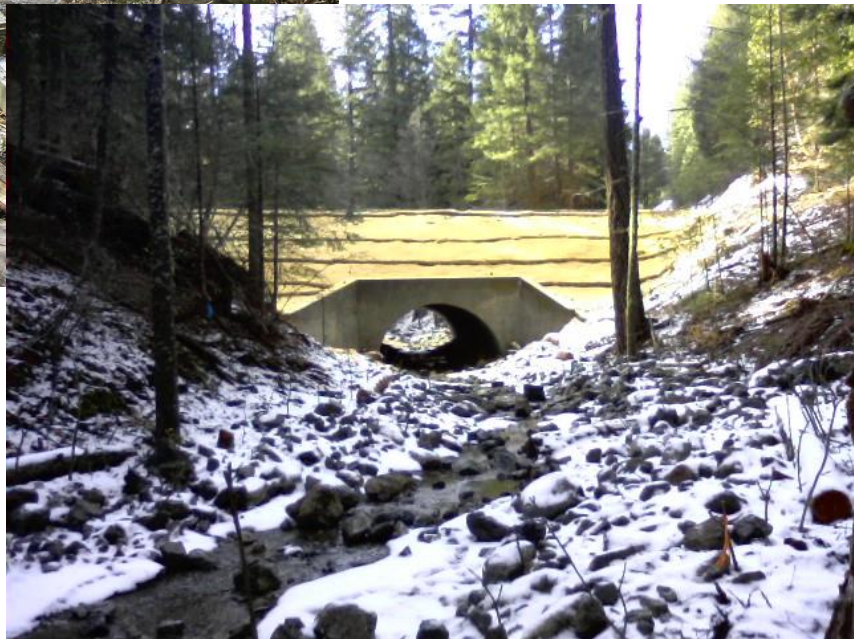
Figure 1: The top photo features an example of a fish barrier that was remediated on the Shasta-Trinity National Forest. The bottom photo features the solution to the barrier—an open-bottom arch composed of natural streambed. This barrier remediation project created newly accessible habitat for Coho Salmon, Klamath Mountain Province steelhead, and Pacific lamprey. Photo credits: Shasta-Trinity National Forest
