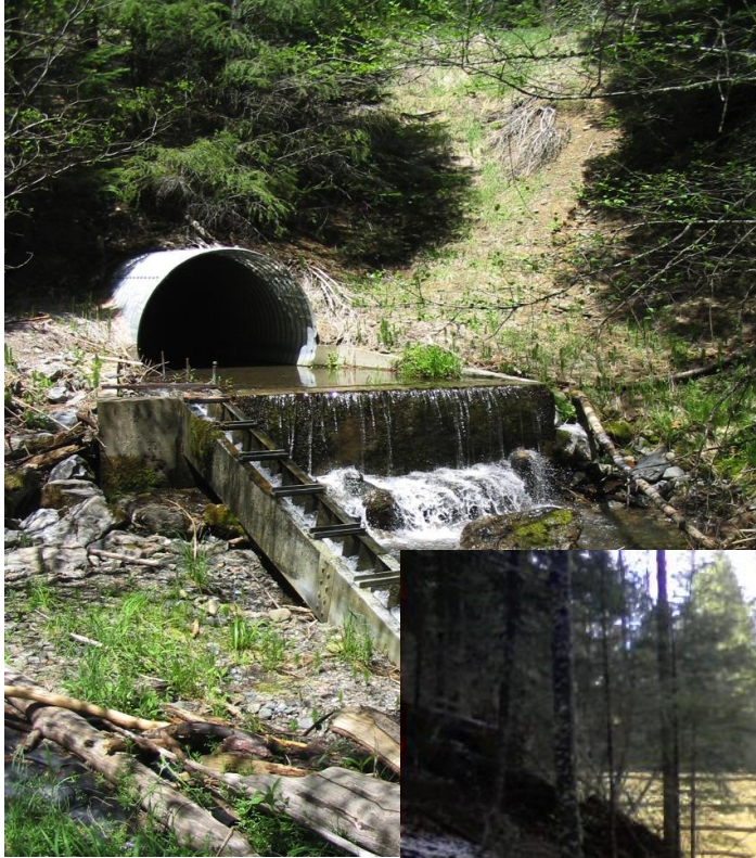
Figure 1: The top photo features an example of a fish barrier that was remediated on the Shasta-Trinity National Forest. The bottom photo features the solution to the barrier—an open-bottom arch composed of natural streambed. This barrier remediation project created newly accessible habitat for Coho Salmon, Klamath Mountain Province steelhead, and Pacific lamprey. Photo credits: Shasta-Trinity National Forest
