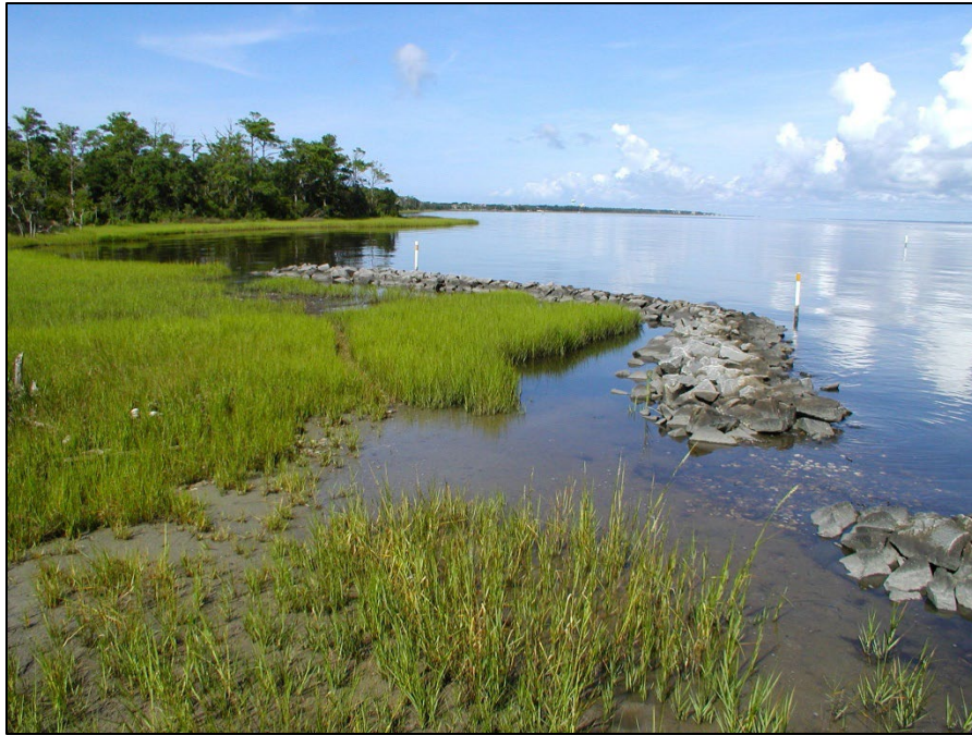
Figure 7 – This living shoreline project will address existing shoreline degradation through the construction of additional structures intended to attenuate waves and attract oyster growth while accompanying marsh plantings will help to stabilize bare areas of marsh platform.
