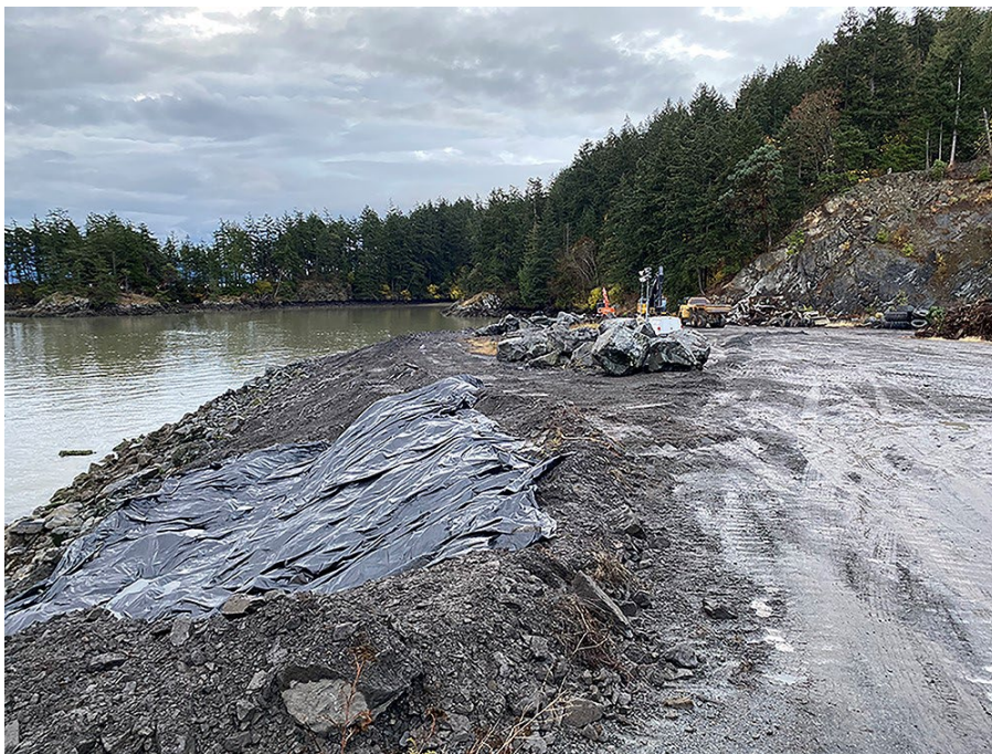
Figure 6 - By removing the armor rock and re-grading the shoreline during its mine reclamation project, the Lummi Island Heritage Trust was able to connect the upland corridor to nearshore habitat and help the shallow water habitat recover its natural processes. Photo Credit: Lummi Island Heritage Trust
