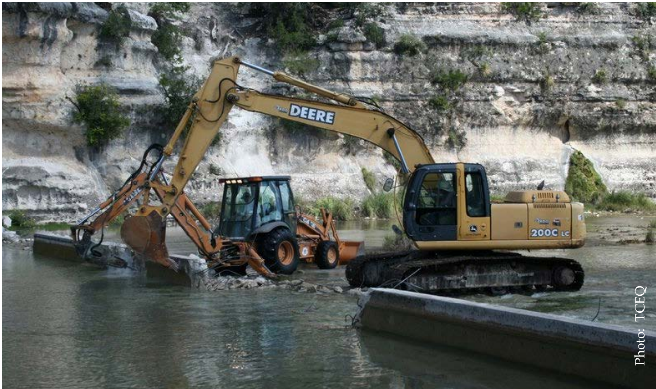
Figure 22 - Dam being removed from the North Fork Guadalupe River located in the Southern Edwards Plateau Rivers Native Fish Conservation Area.
